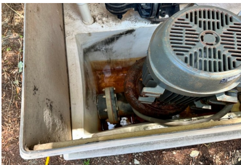
Slide Pool Pump in Need of Repairs & Sump pump replacement
