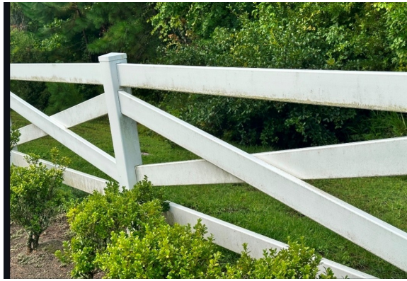
Vinyl Fencing Pressure Washed
