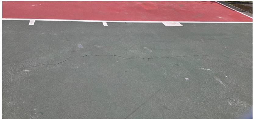
Area Of Concern: Large Cracks in the Basketball Court Foundation –
