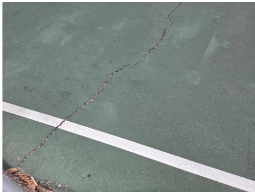
Area Of Concern: Large Cracks in the Basketball Court Foundation –
