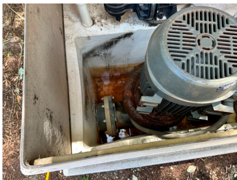
Slide Pool Pump in Need of Repairs & Sump pump replacement
