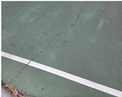
Area Of Concern: Large Cracks in the Basketball Court Foundation –
