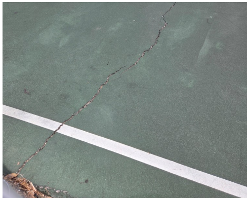
Area Of Concern: Large Cracks in the Basketball Court Foundation –
