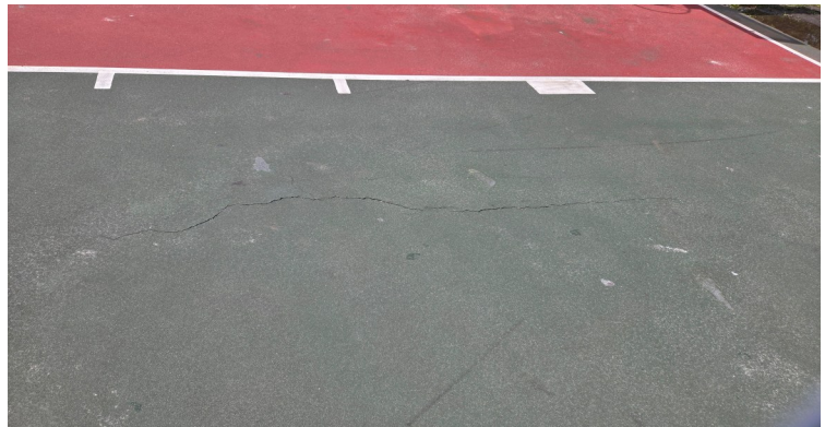
Area Of Concern: Large Cracks in the Basketball Court Foundation –
