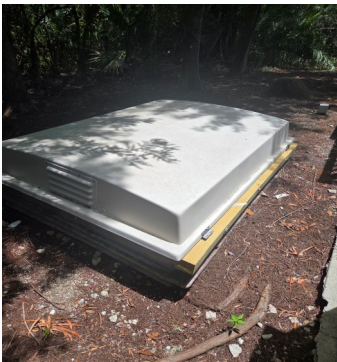
Slide Pool Tank Repaired
