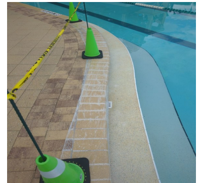
Pavers & Coping Repaired by Lap Pool Cabana
