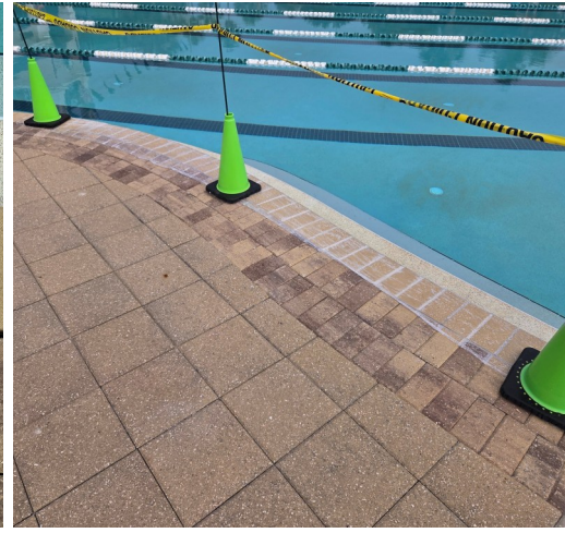
Cracked & Loose Pavers Repaired and Reset
