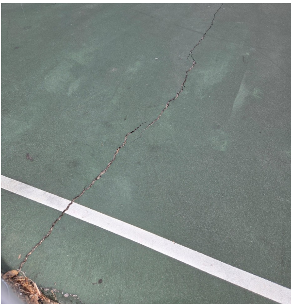
Area Of Concern: Large Cracks in the Basketball Court Foundation
