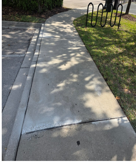
Sidewalk with raised edges and tripping hazard repaired
