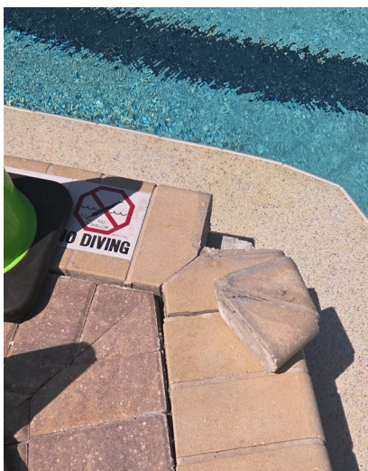
Area Of Concern: Pool Ledge Pavers are Loose - Update Repaired
