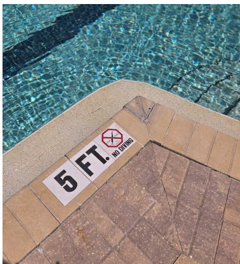
Area Of Concern: Pool Ledge Pavers are Loose - Update Repaired
