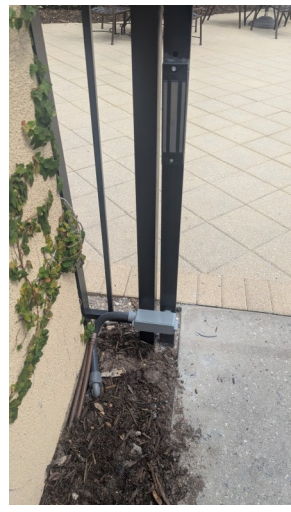
Magnet and Wiring Replacement on Back Pool Gate
