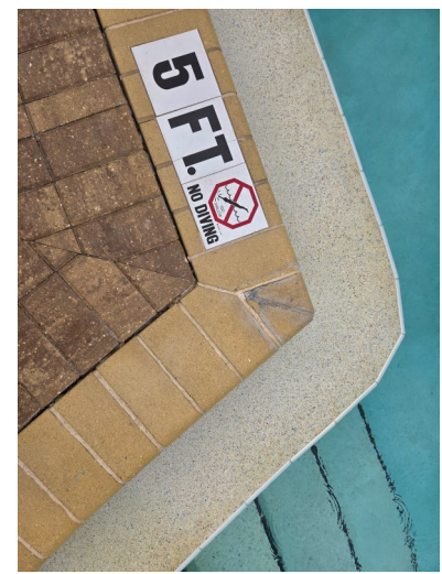
Area Of Concern: Pool Ledge Pavers are Loose - Update Repaired
