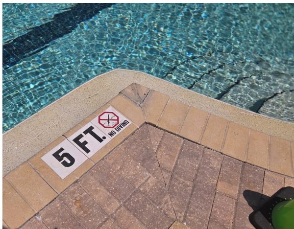
Area Of Concern: Pool Ledge Pavers are Loose
