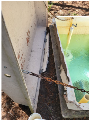
Broken Lid and Fiberglass on Slide Tank in Need of Repair– IN PROGRESS –NEW LID ORDERED
