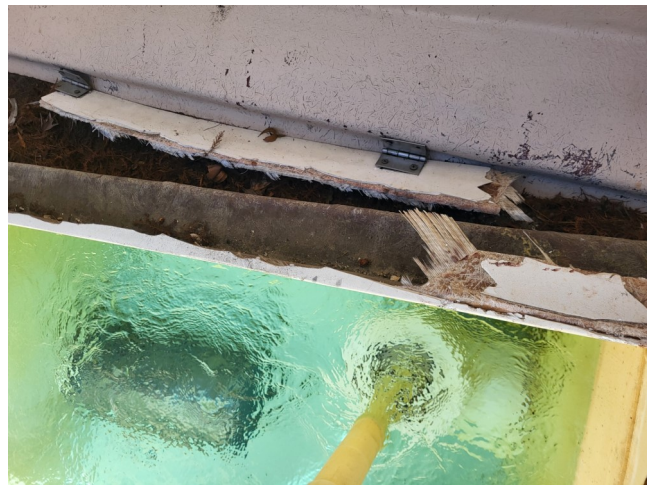
Broken Lid and Fiberglass on Slide Tank in Need of Repair– IN PROGRESS –NEW LID ORDERED
