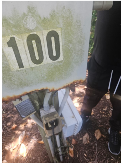
Rusted Electrical Panels Need Replacement - Highland Court, Wellington Park
