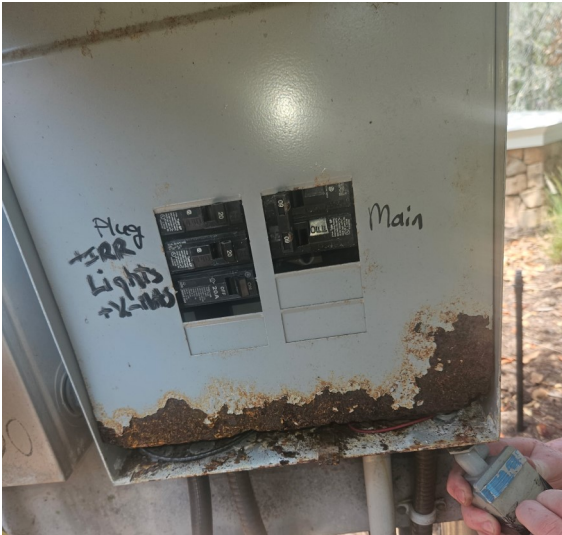
Rusted Electrical Panels Need Replacement - Highland Court, Wellington Park
