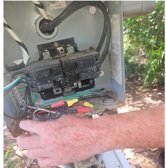
Rusted Electrical Panels Need Replacement - Highland Court, Wellington Park
