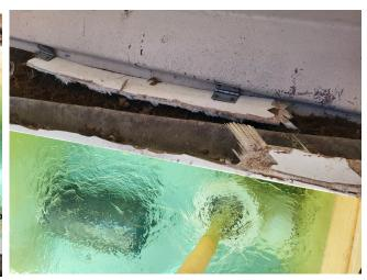
**Broken Lid and Fiberglass on Slide Tank in Need of Repair- IN PROGRESS**
