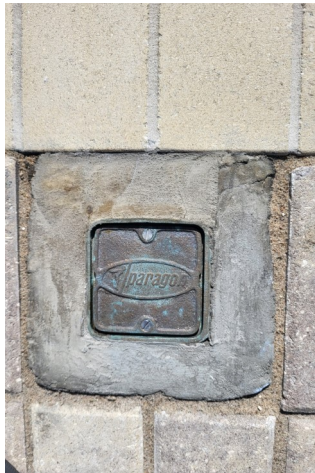
New Dive Block Anchors
