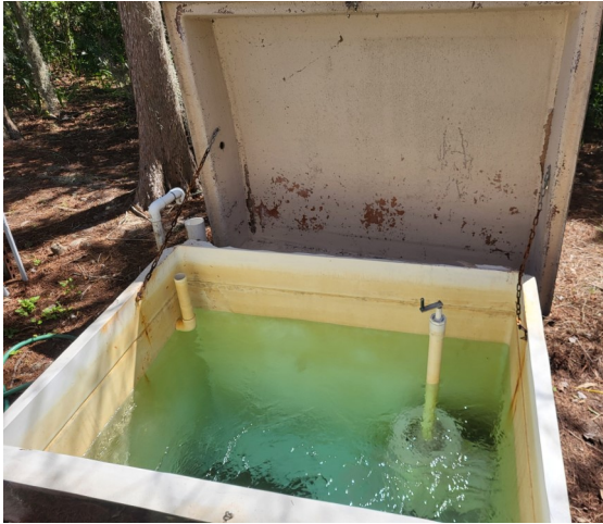
Broken Lid and Fiberglass on Slide Tank in Need of Repair– IN PROGRESS
