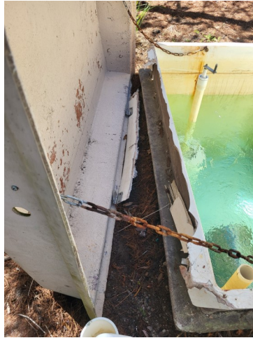
Broken Lid and Fiberglass on Slide Tank in Need of Repair– IN PROGRESS
