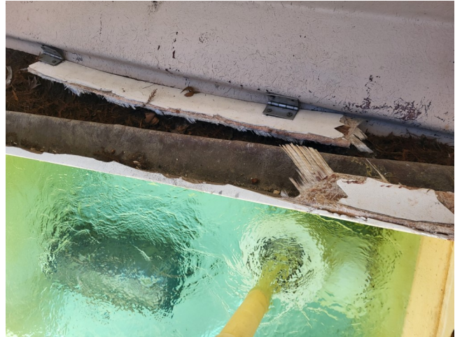
Broken Lid and Fiberglass on Slide Tank in Need of Repair– IN PROGRESS
