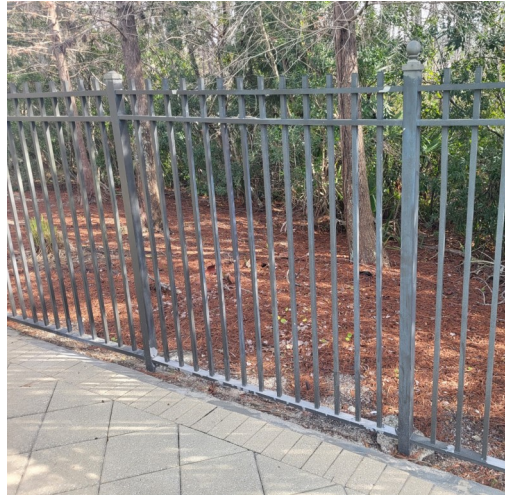
Existing exterior Amenity Center Fencing in need of repainting
