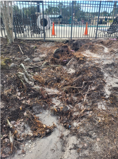
Washout due to broken reclaimed water line and old Cypress roots.
