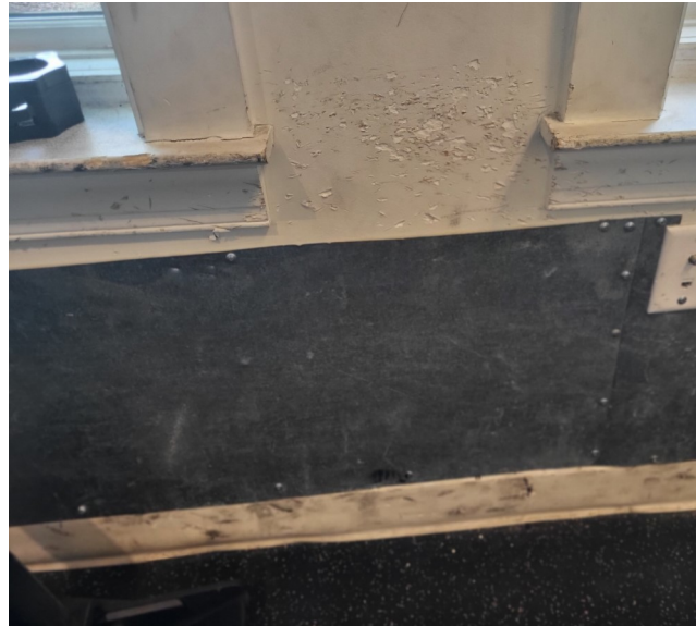
Repairs, Painting and Replacement of Aluminum Sheeting Required in Fitness Center
