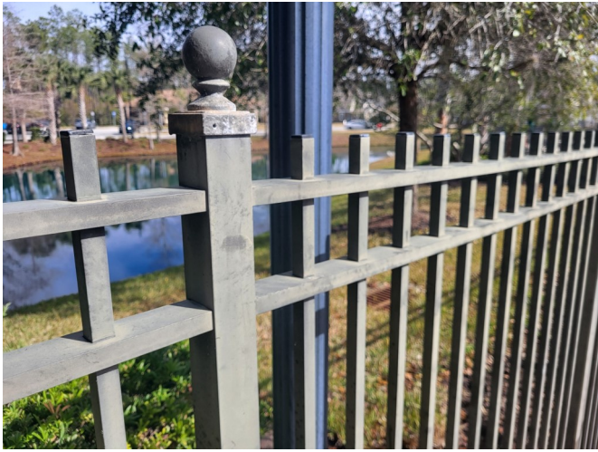
Existing exterior Amenity Center Fencing in need of repainting
