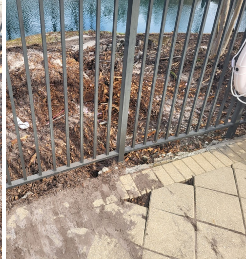
Washout due to broken reclaimed water line and old Cypress roots.
