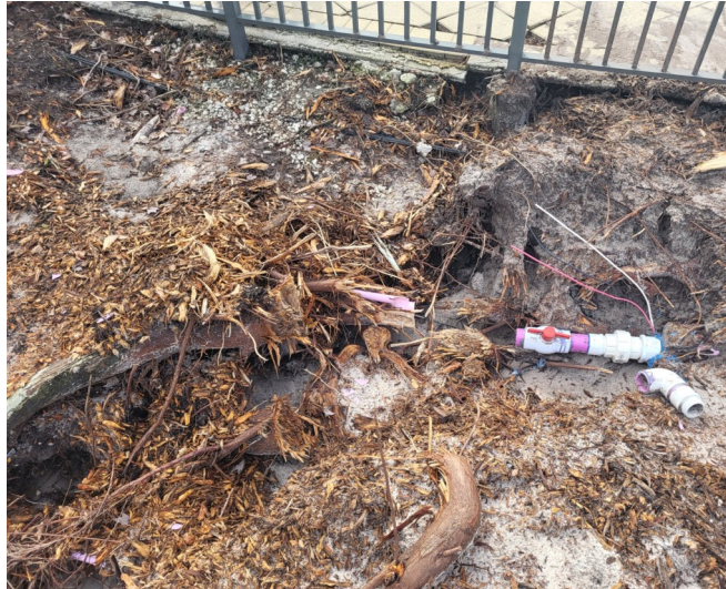
Washout due to broken reclaimed water line and old Cypress roots.
