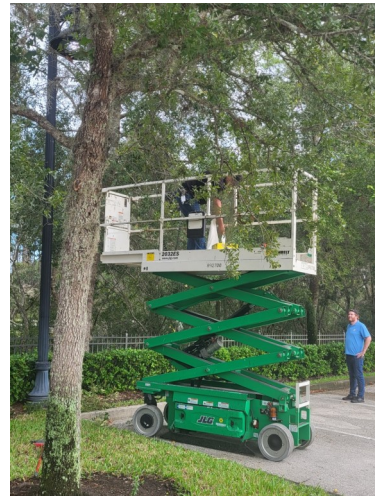
Parking Lot Lights Repaired—Lift Required
