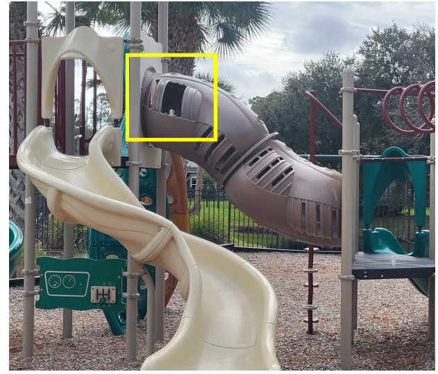
Broken Slide—Replacement Part Ordered
