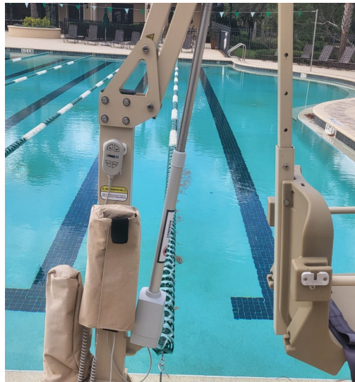
ADA Chair Actuator Replaced
