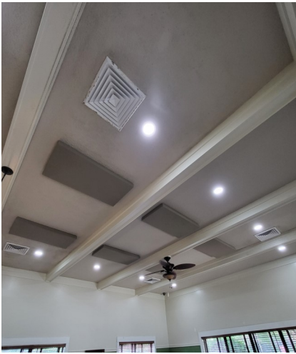
SH Replaced with LED Lights
