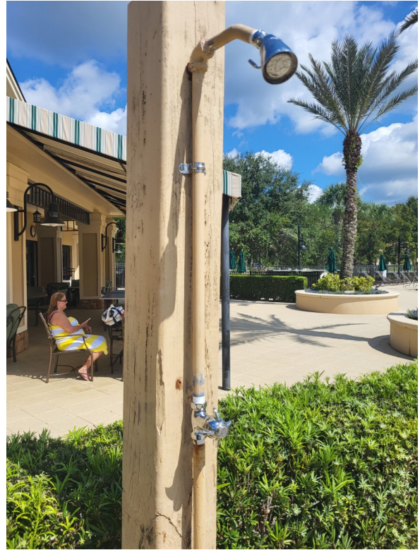
Pool Shower Handle Replaced
