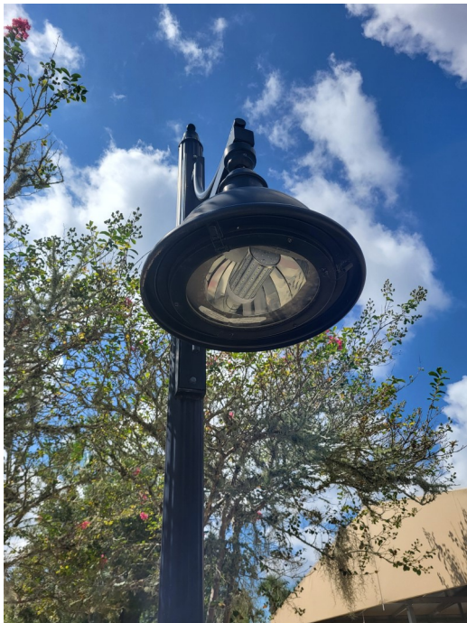
Pool Deck Lights Replaced
