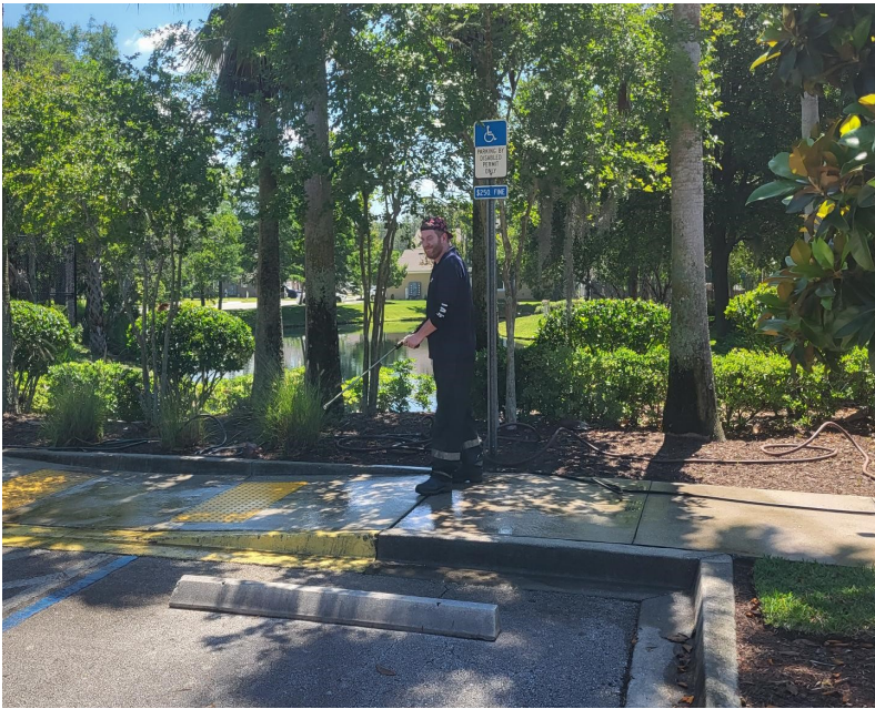
Sidewalk pressure washed
