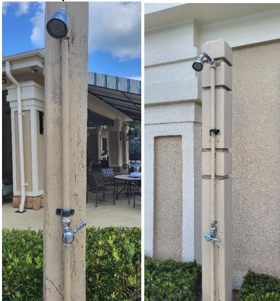
Replaced Shower Handles
