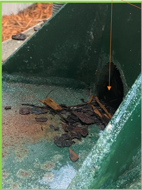
Rust appearing from Drain Ports:
