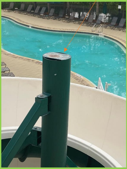
Rust appearing from Drain Ports:
